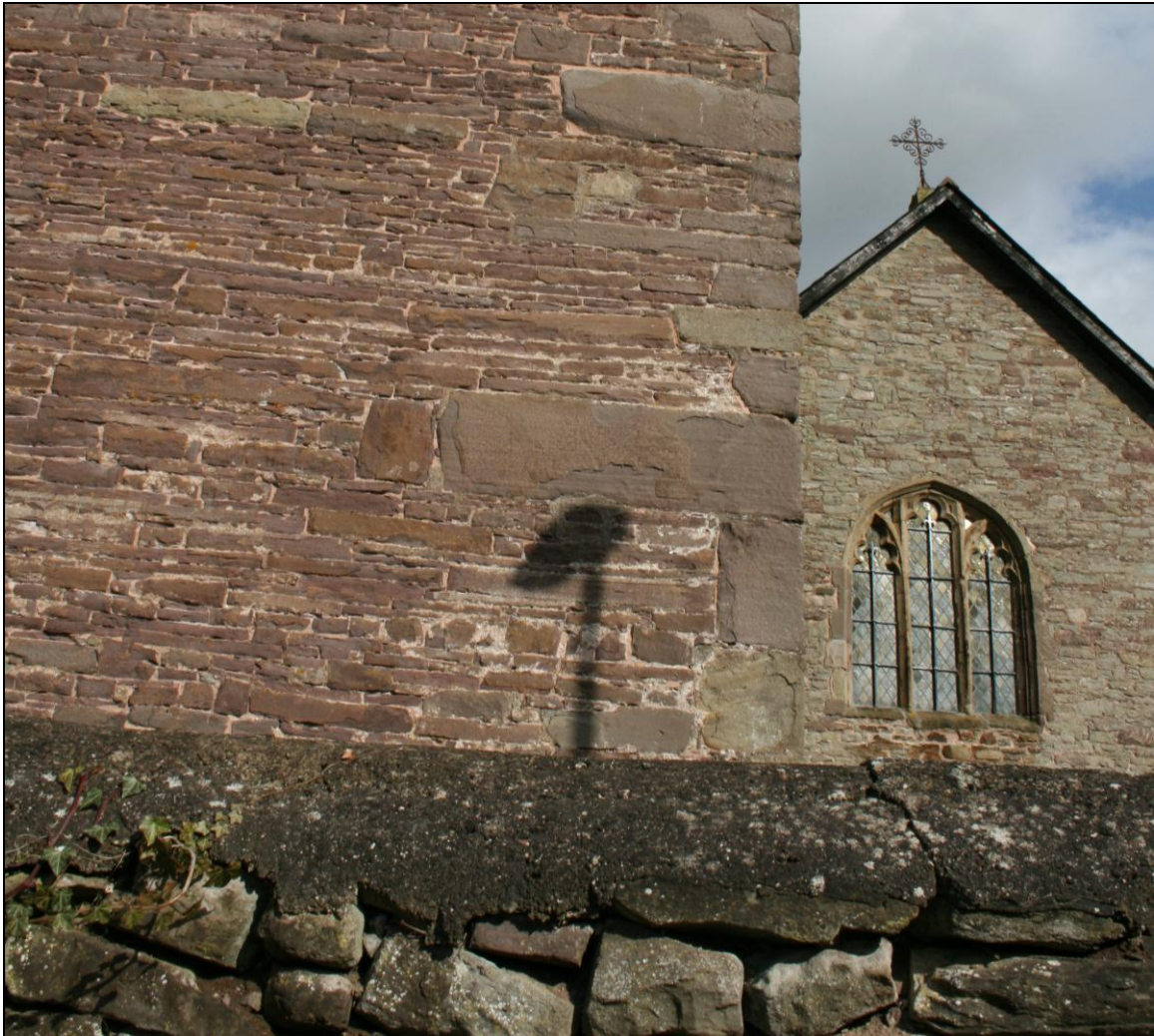
Differing sandstone colours and details on the Parish Church
