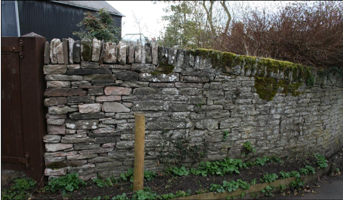
Roughly coursed and dressed walling with vertical coping
