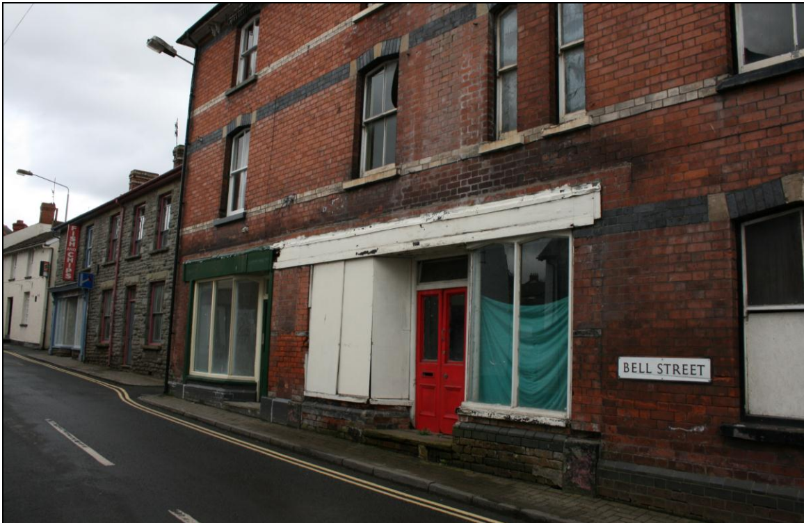
Problems with former commercial premises, Bell Street
