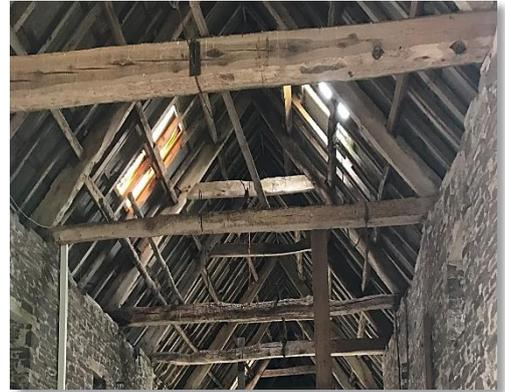
3.6.28 Interior heights of rural buildings may be too restricted to allow for two floors. If adequate headroom cannot be achieved on the first floor, the design of the conversion should be revisited instead of cutting the roof trusses.
