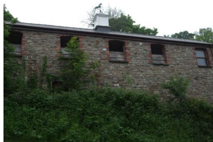
Neglected industrial building alongside former railway line.
