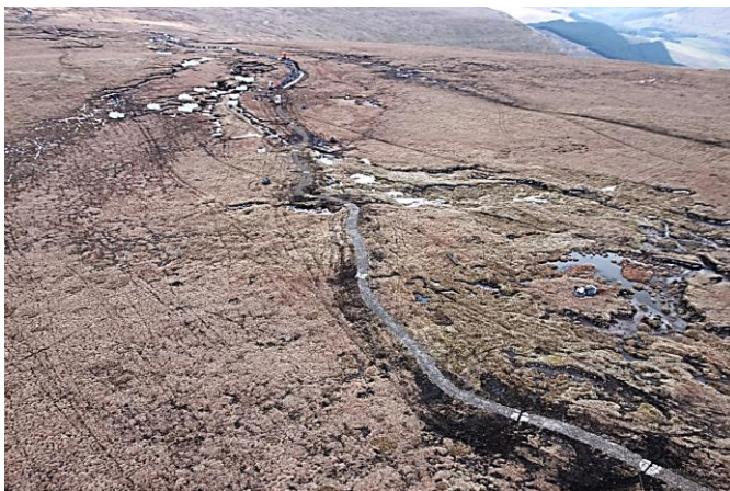
Footpath construction to repair and reduce widespread erosion across peat
