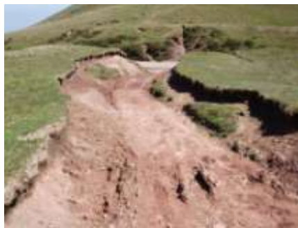
Footpath erosion (Gospel Pass)
