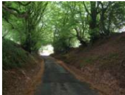
Damage to hedgebanks on narrow lanes caused by wide or passing vehicles.
