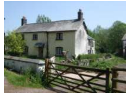
Locally distinctive farmhouse in a poor state of repair
